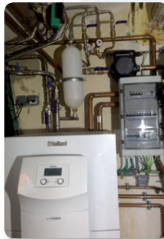
installation of an air to water heat pump, the geoTHERM VWL 171/3 S model from Vaillant. The annual cost of this model is less than other systems, offers improved energy certification by achieving a B rating, needs very little space, with no need for a chimney and is the cleanest option available as it does not need combustible fuel. The initial investment would be slightly higher, however would be amortised in the medium-term.
